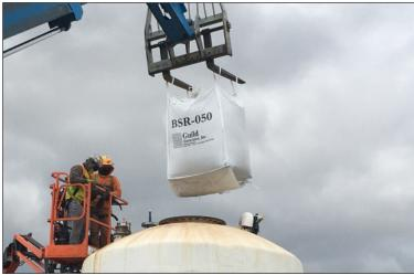
BSR-050 from Guild Associates is a high-capacity granular media for the removal of hydrogen sulfide from biogas. Engineered for direct replacement of Iron Oxide and Activated Carbon media in dry media systems, BSR-050 is field-proven to treat bopgas gas for power generation and Renewable Natural Gas.
