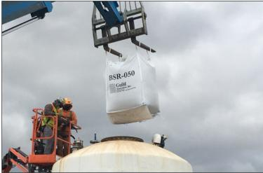
BSR-050 from Guild Associates is a high-capacity granular media for the removal of hydrogen sulfide from biogas. Engineered for direct replacement of Iron Oxide and Activated Carbon media in dry media systems, BSR-050 is field-proven to treat biogas gas for power generation and Renewable Natural Gas.
