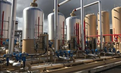
Guild Associates' Molecular Gate  $CO_2$  Pressure Swing Adsorption system offers high methane capture efficiency and low operational costs. Standard features include:
