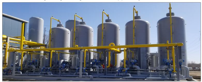
Landfill gas is usually contaminated with carbon dioxide, nitrogen and oxygen, each requiring unique molecular separation technologies. Guild Associates has developed the Equilibrium Pressure Swing Adsorption (PSA) system, which can operate downstream from virtually any CO<sub>2</sub> removal technology to remove the nitrogen and oxygen to pipeline quality levels.
